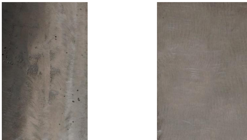
Fig.3. Blow hole and Grinding defect
